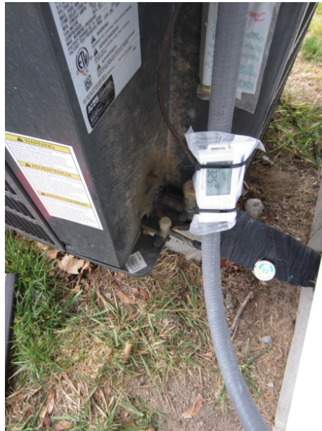
Figure 1. Installation of run-time logger
