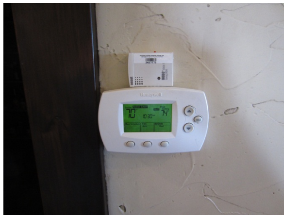
Figure 2. Installation of Thermostat Logger
