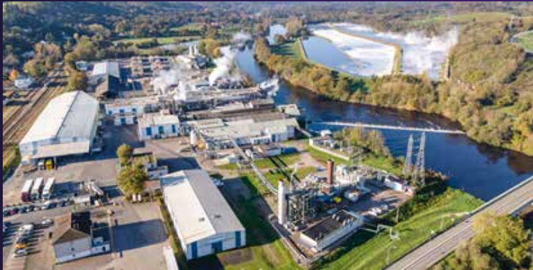
Smurfit Kappa SGT-400 Cogeneration Plant Saillat-sur-Vienne, France
