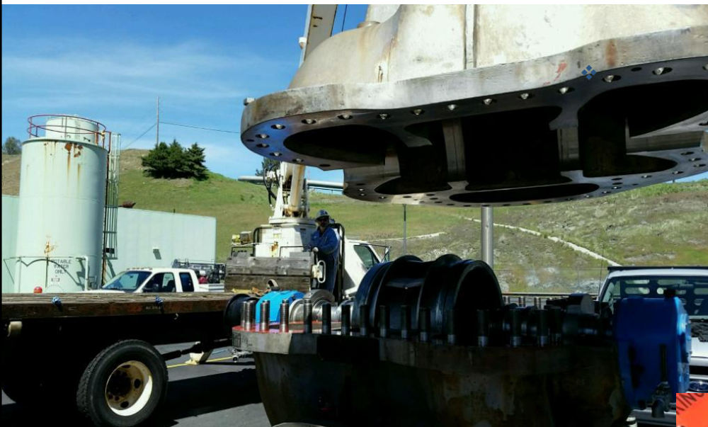
NCPA GEO Team pulling the top off the pump
