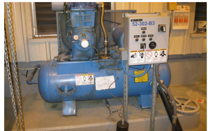
Air Compressor for Surge Tanks
