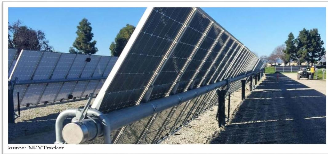
Figure 2.3-4 Typical HSAT PV Array with Bifacial Modules
