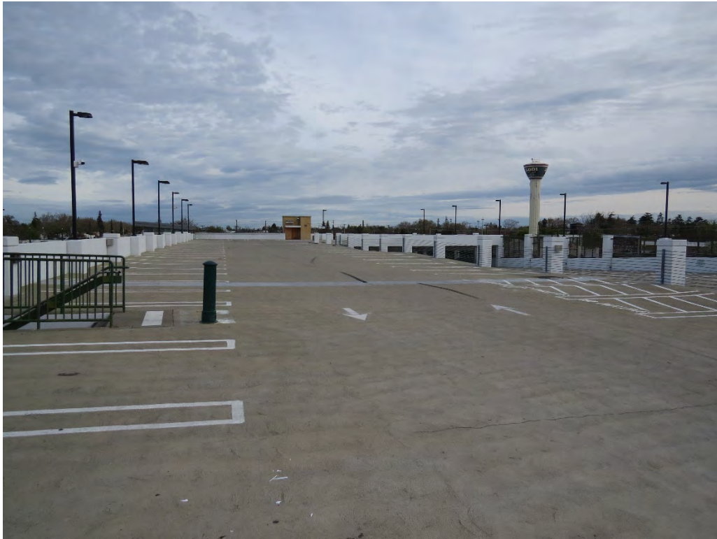
Photograph 1: From the southwest corner of the Parking Garage site looking north.
