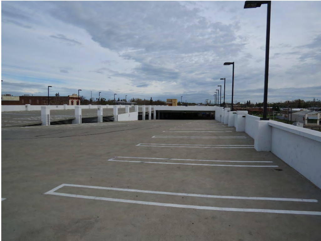
Photograph 3: From the southeast corner of the Parking Garage Site looking northwest.
