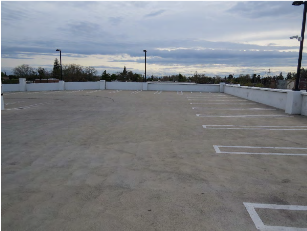
Photograph 2: From the southwest corner of the Parking Garage site looking east.
