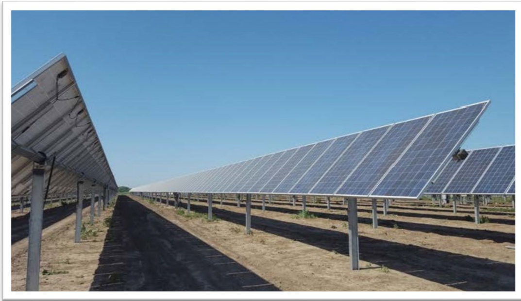
Figure 2.3-3 Typical Fixed Tilt Solar Array
