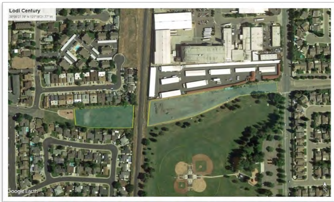
Figure 2 Century Park East/West Site
