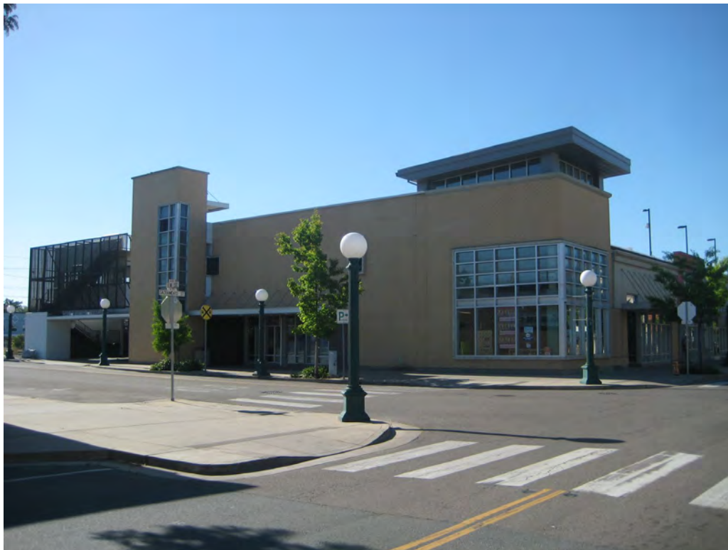
Photograph 3. North elevation of parking garage, facing south-southeast.
