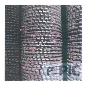
Fig 1.0 HRSG tubes before cleaning
