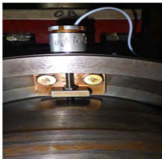
Generator vibration probe mounting (Top center)
